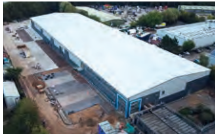
New manufacturing and operational centre in Bury St. Edmunds, UK.
